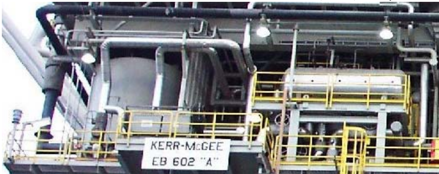
Uniflux heater and Pump Skid: This is a close-up of the left side of the cover photo. This unit has been in service since 2002.
